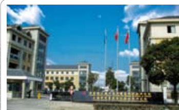
2011 Shanghai Institute of Quality Inspection and Technical Research
